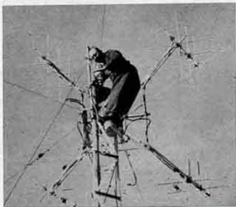
Up goes the 4-bay tracking antenna at W6EE. W6ASH balances atop the 30-foot tracking tower on the roof of the Project Oscar building. The cross-polarized array is rotatable and movable in elevation.
